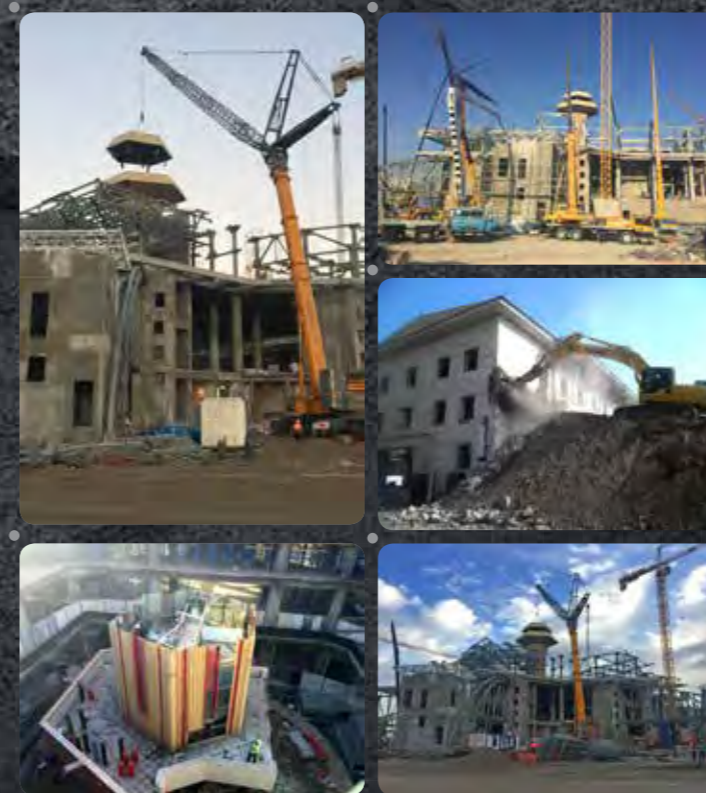
Ashgabat International Airport – Demolition and dismantling works AŞGABAT 2013- 2015
